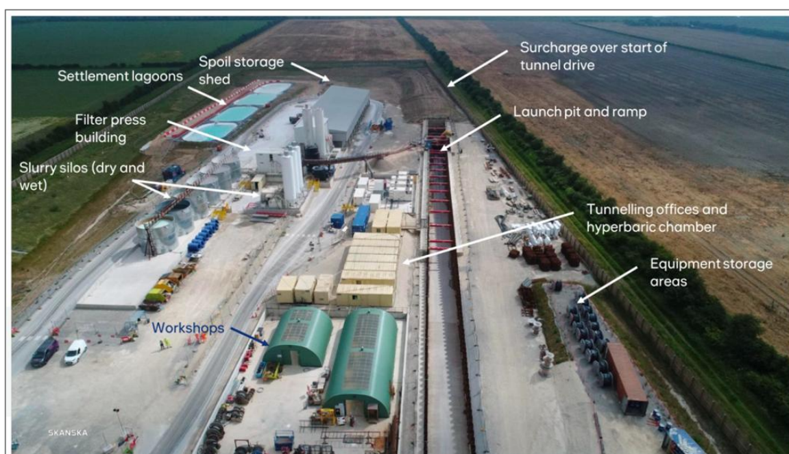
Figure 9 Representative tunnel set up – NGV Feeder 9 Project
